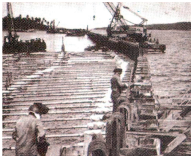
The construction of a wharf
