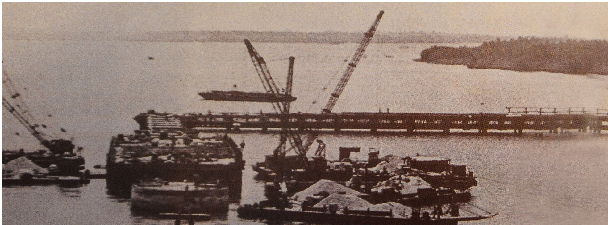
The construction of oil jetty
