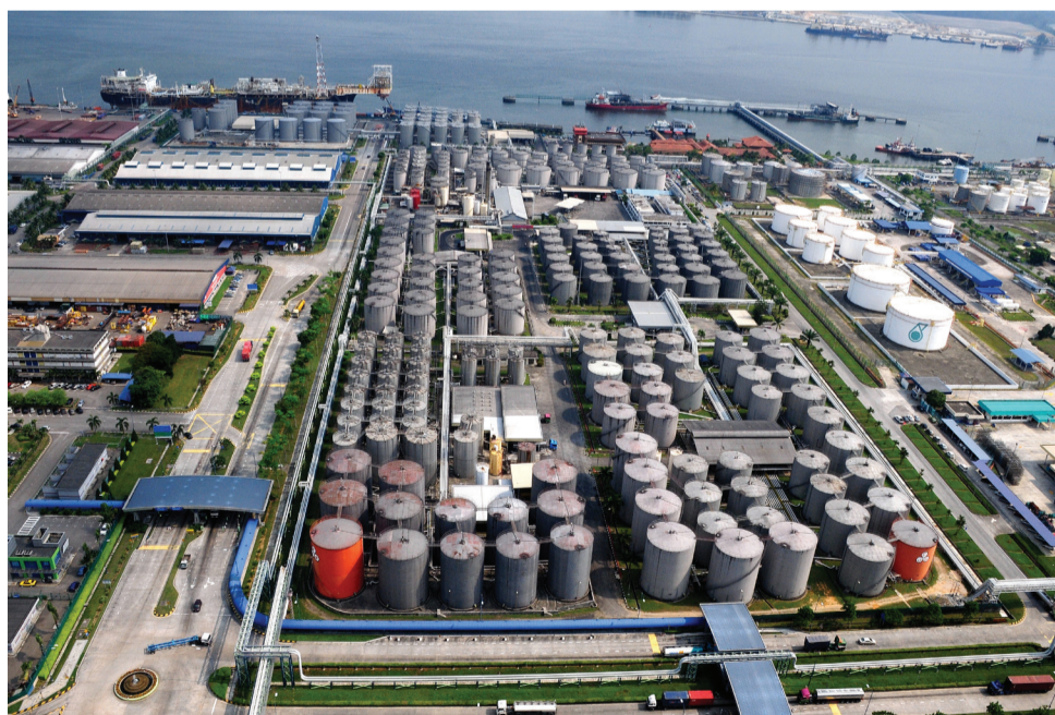
Johor Port's tank farm for edible and non-edible liquid has the capacity of storing 1 million metric tonnes
